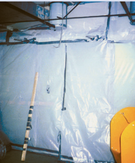
Photo 8: Full containment on large job
